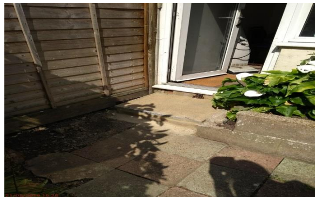
Condition at final inspection
