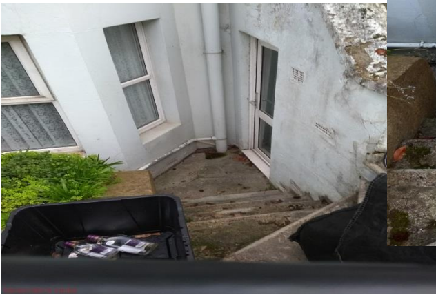
Condition at Initial Inspection
