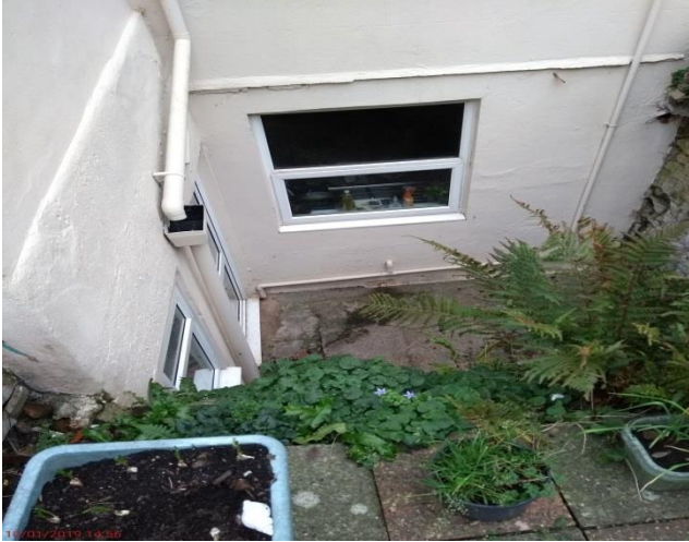
Condition at initial inspection
