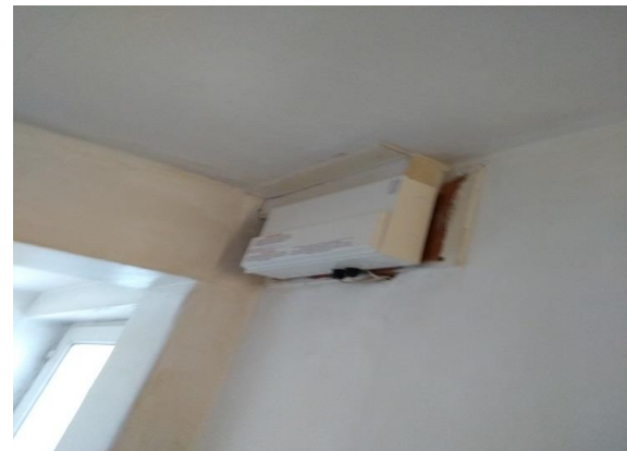
Condition at final inspection
