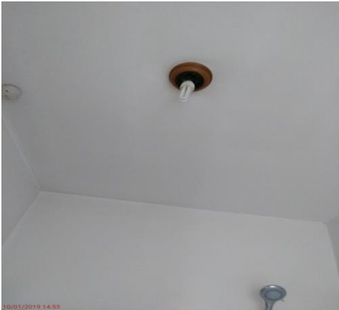
Condition at final inspection
