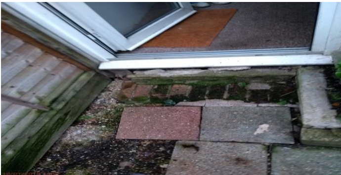
Condition at initial inspection
