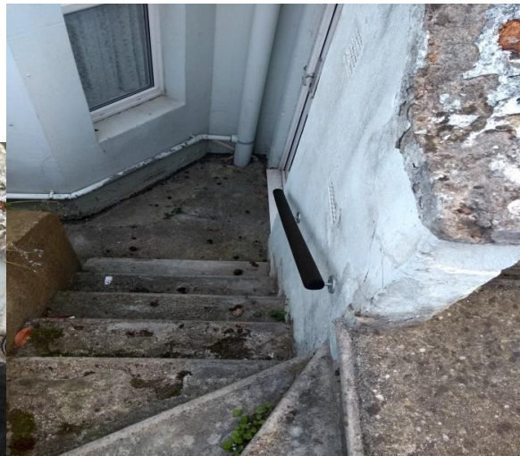
Condition at final inspection
