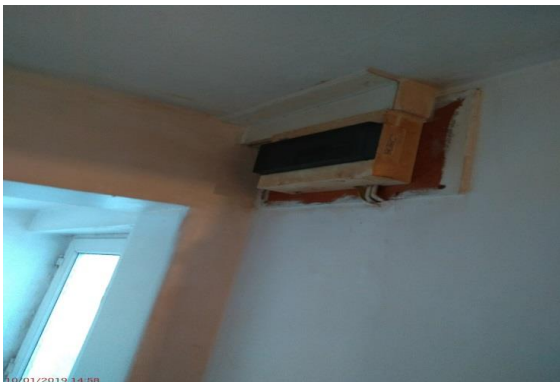
Condition at initial inspection
