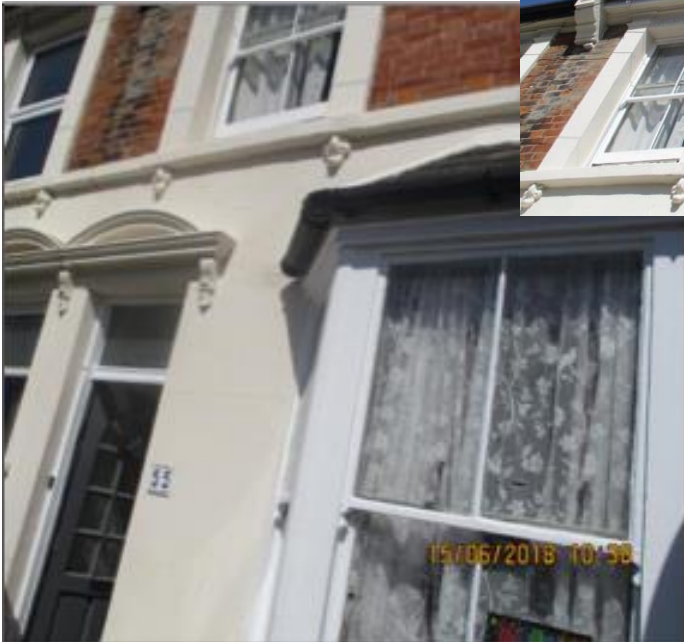
Front elevation after work (above and left)
