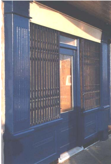
Security gate integrated into the shopfront
