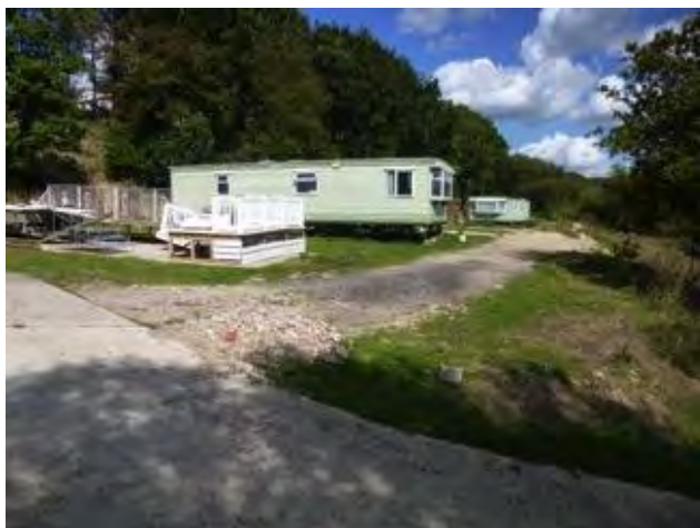
Lower section affected by landslip 73 and 74
