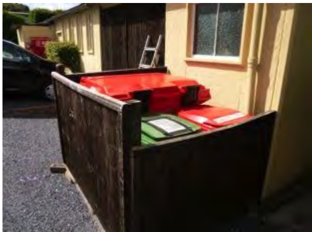
Refuse Point at Workshop
