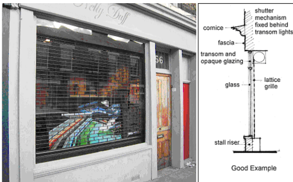
Photo showing an acceptable 'open' shutter that allows the inside of the shop to be seen and does not mask the detail of the shopfront
