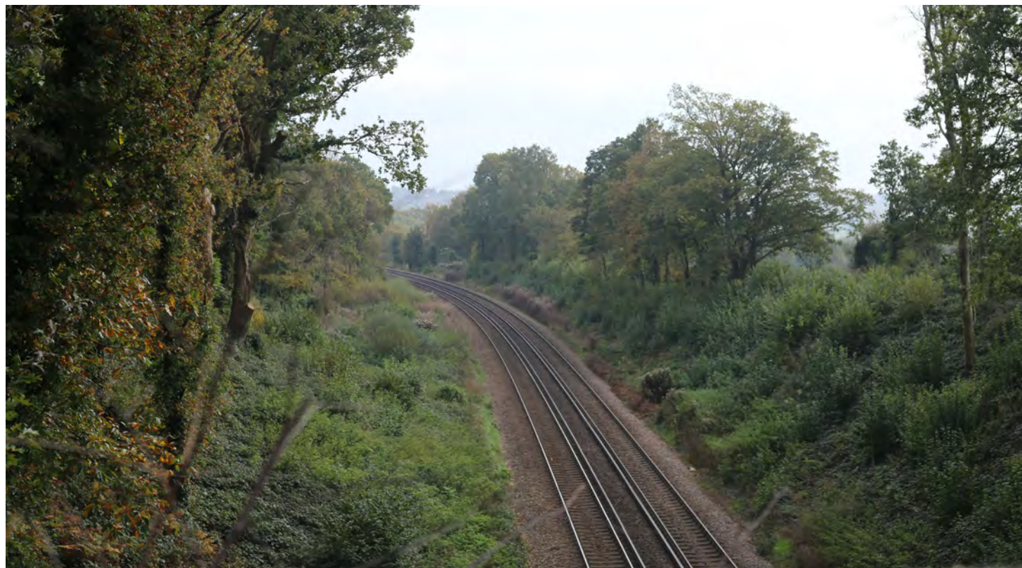
LCCA1 - Context Photograph 1C. The London to Hastings Railway extends variously within a cutting or part raised embankment, defining the north-eastern edge of the Combe Valley Countryside Park.
