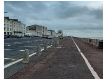
Along sea front Compartment 99 (TQ 79877 08797)
