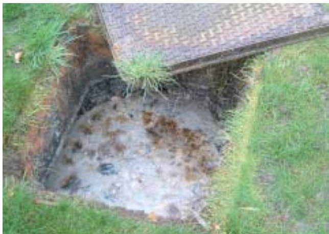
Fat building up in a manhole
