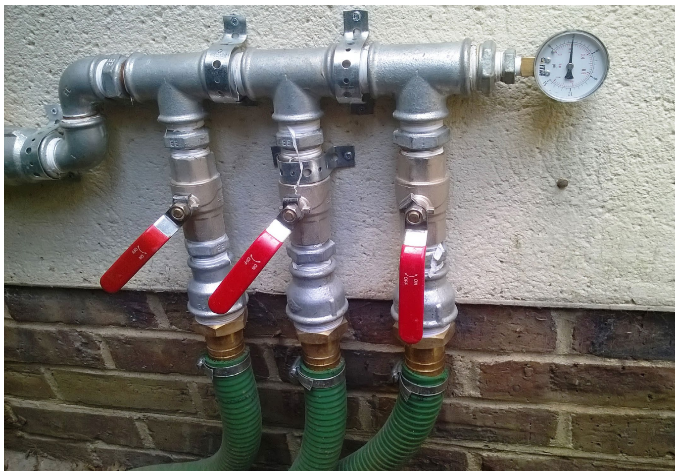
Compressor arrangement - showing standard position of levers and pressure
