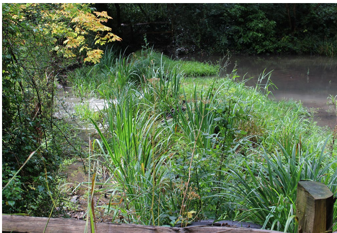
Vegetated bund to encourage silt deposition
