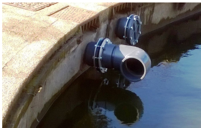
Overflow Pipes
