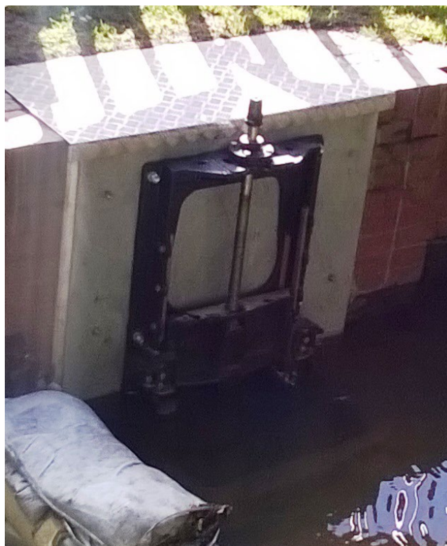
Penstock in closed position
