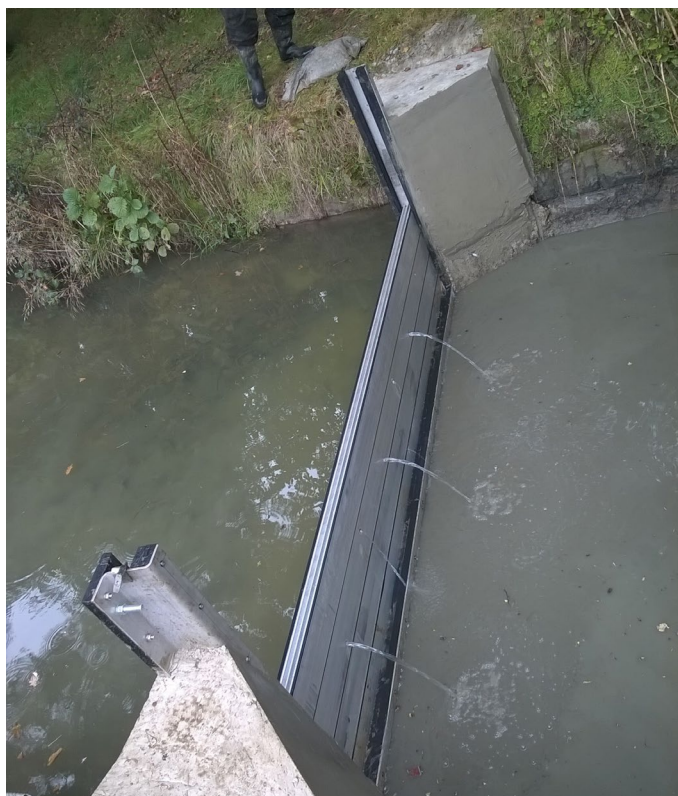
Stop logs showing removed bolts and free flow of water
